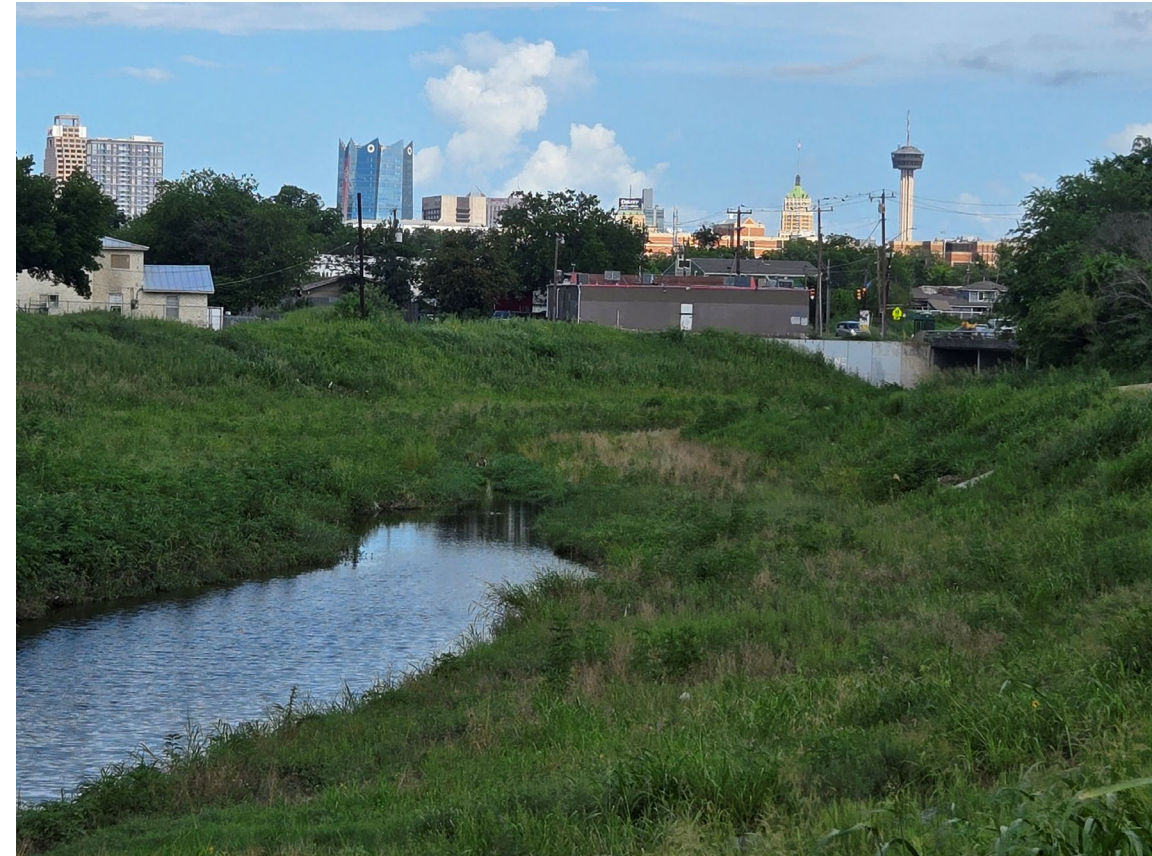
Alazan Creek Looking east down stream West of W. Martin St.
