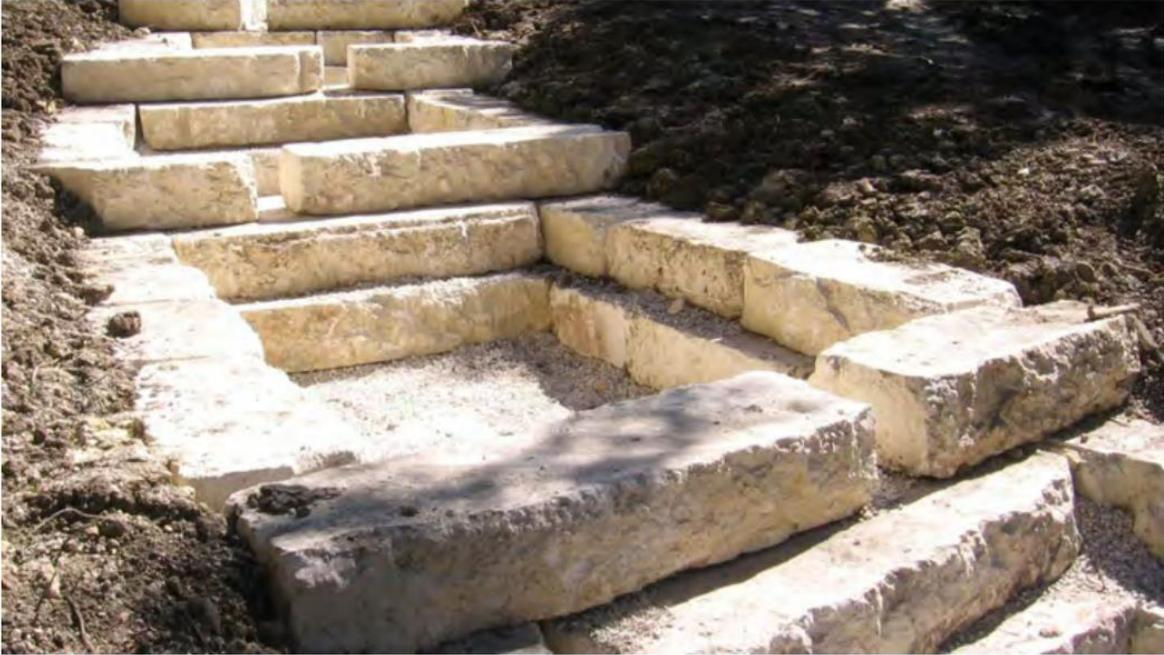
Figure 14. Example of Constructed Step Pools Using Native Central Texas Material (Limestone Blocks) at a Storm Sewer Outfall
