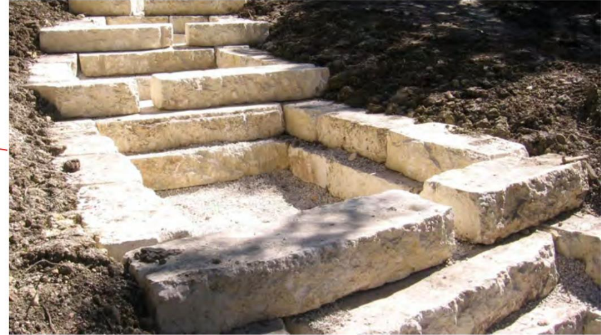
Figure 14. Example of Constructed Step Pools Using Native Central Texas Material (Limestone Blocks) at a Storm Sewer Outfall
