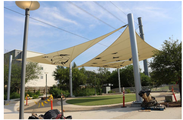
The shade structure has been installed.
