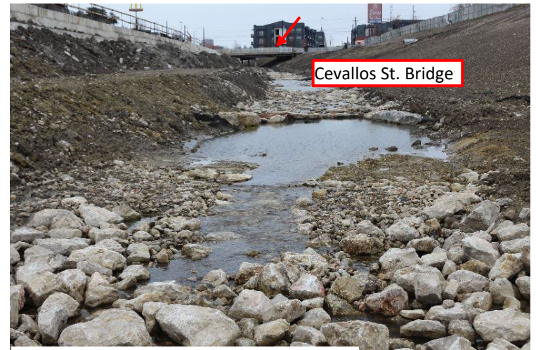
Phase 3 Channel as seen facing north.
