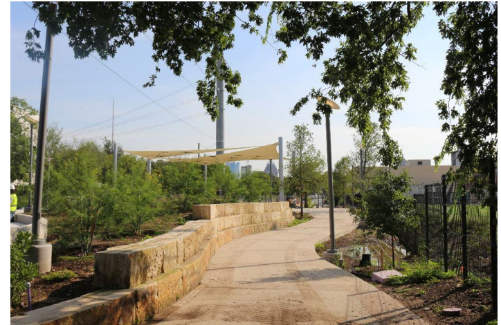
Two of the shade structure Panels have been installed.
