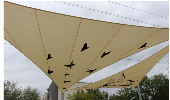
Two of the shade structure Panels have been installed.
