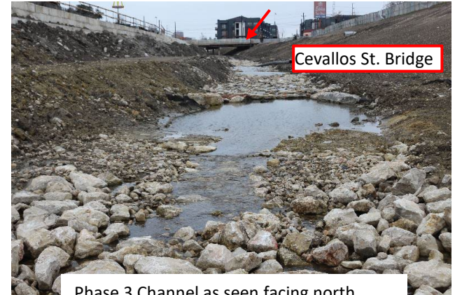
Phase 3 Channel as seen facing north.
