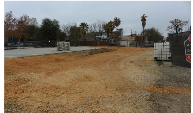
Phase 4.1 As seen from the northwest corner of the parking lot.
