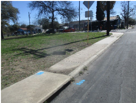
Painted marker for ground survey
