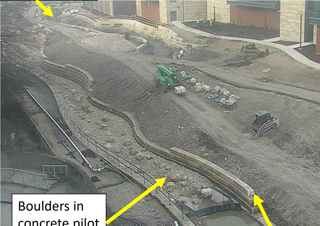
Bioretention pond
