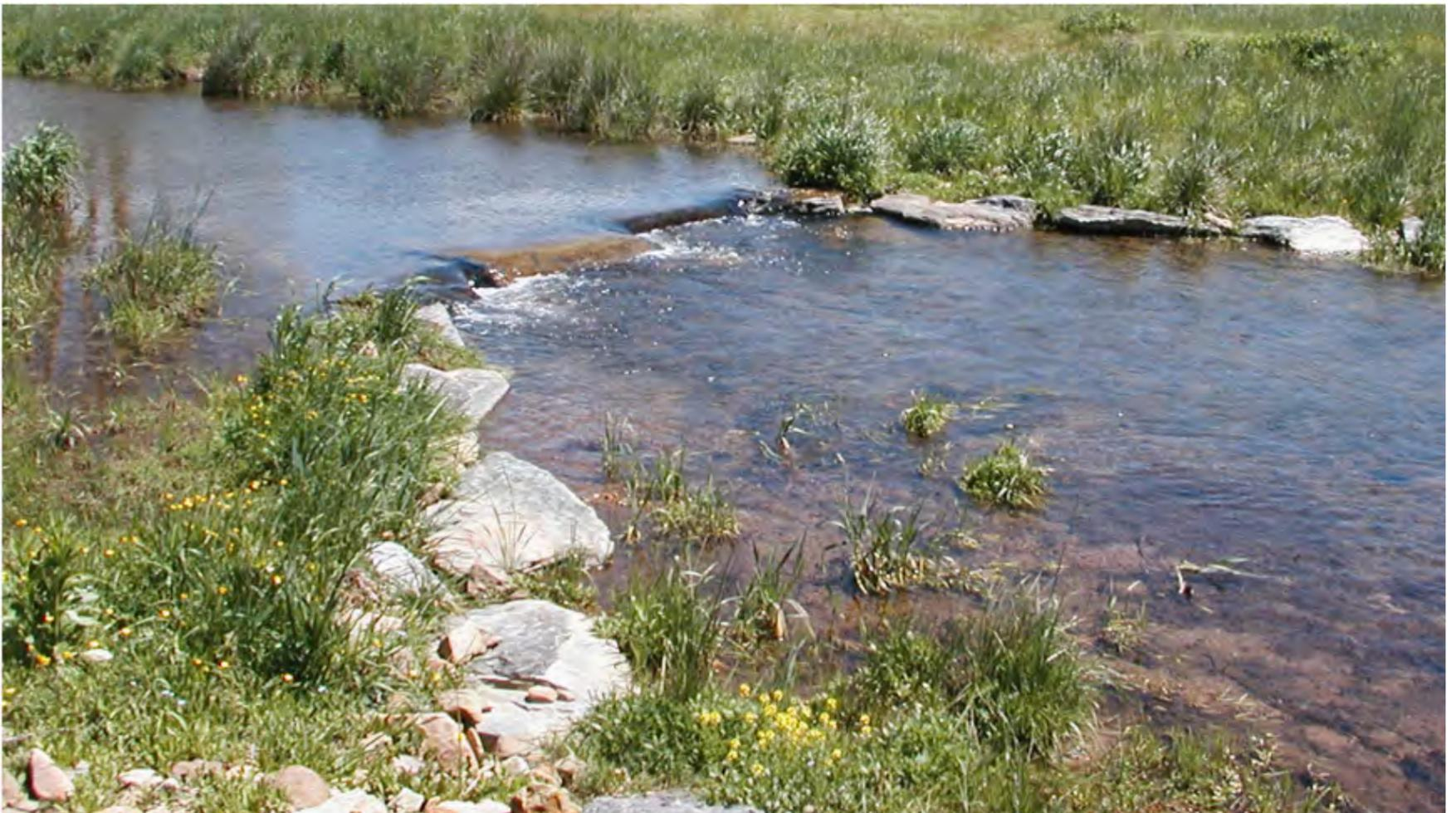
Figure 12. Example of a Constructed Rock Cross Vane
