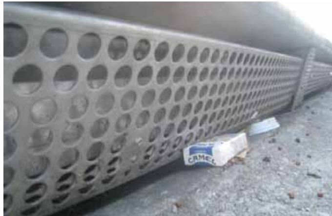
Figure 6.7: Catch Basin Screen Cover
