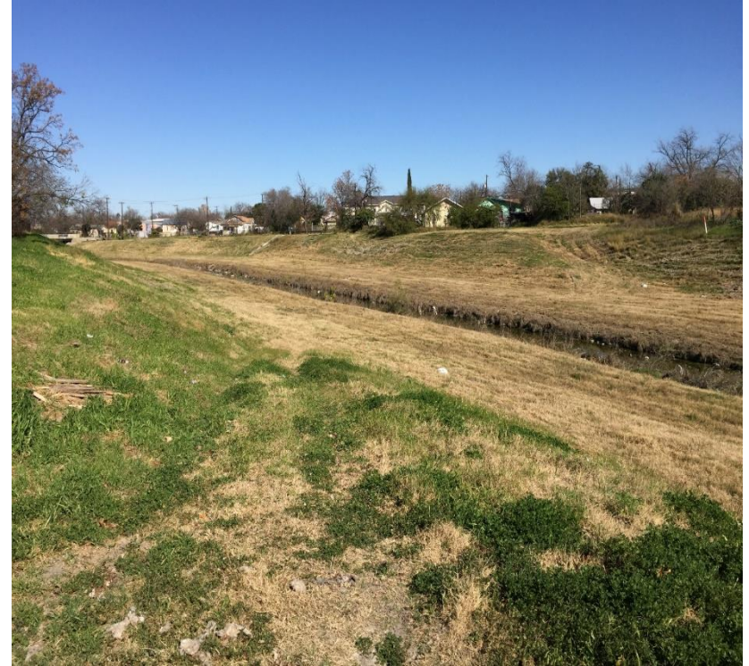
Alazan Creek Looking Upstream
