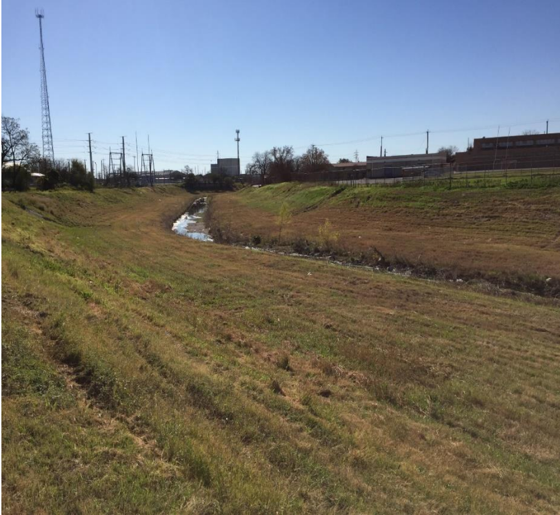
Alazan Creek Looking Downstream
