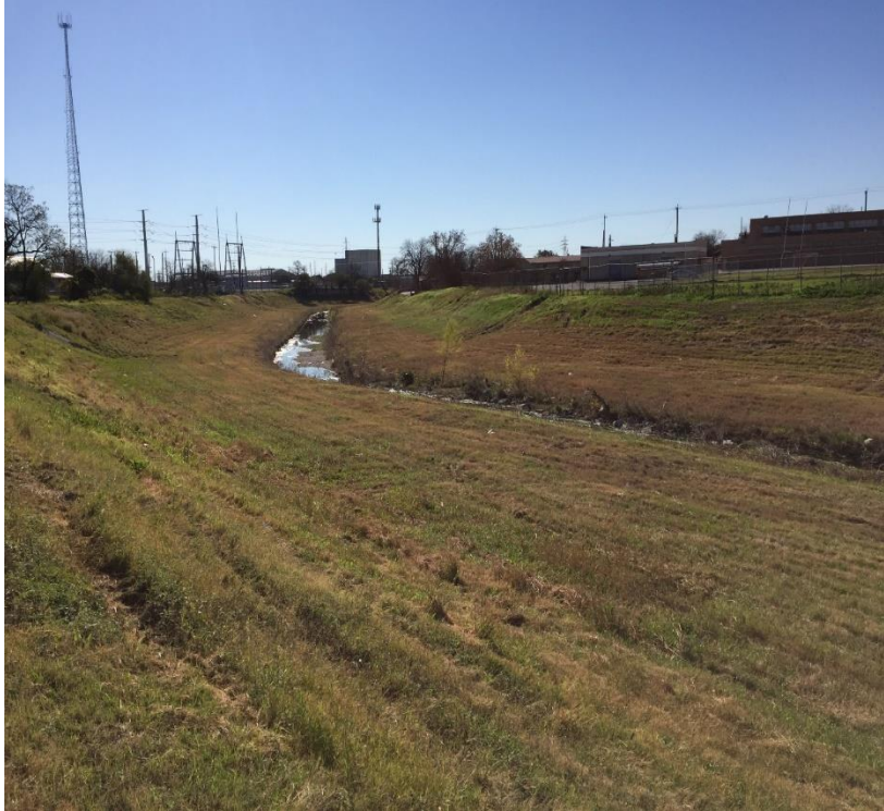
Alazan Creek Looking Downstream
