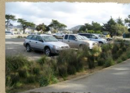
Bioswales purify water and keep excessive water from reaching Cibolo Creek and causing flooding.
