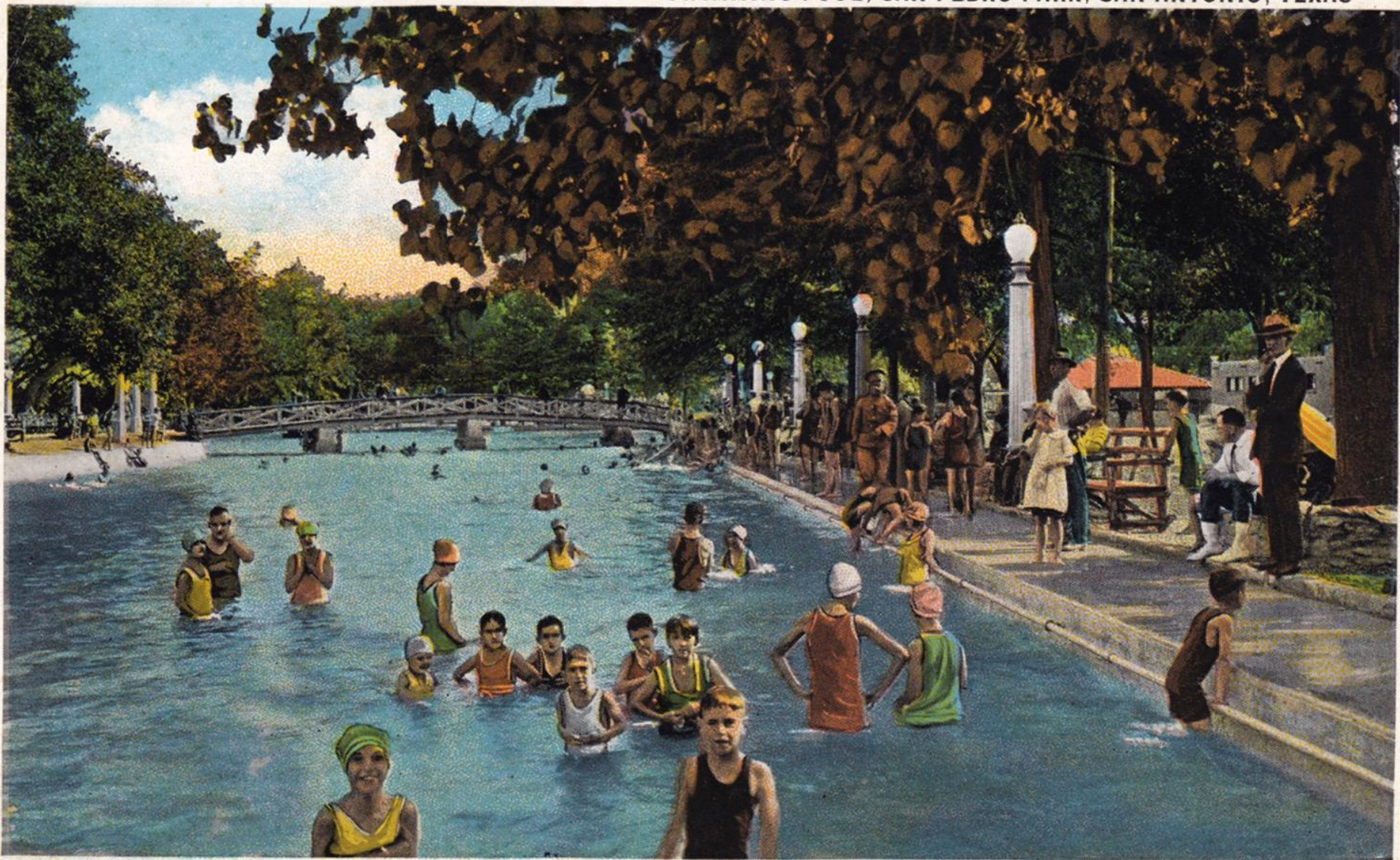
SWIMMING POOL, SAN PEDRO PARK, SAN ANTONIO, TEXAS
