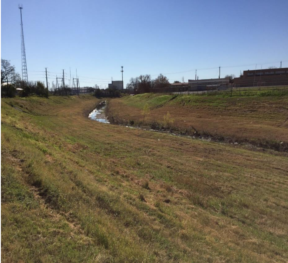
Alazan Creek Looking Downstream
