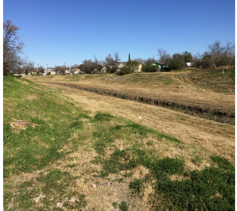
Alazan Creek Looking Upstream
